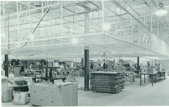
The plant in Ronkonkoma, New York, was built in 1980 and the square footage doubled the following year.
