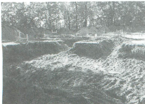
The preparation for foundation footings begins.
